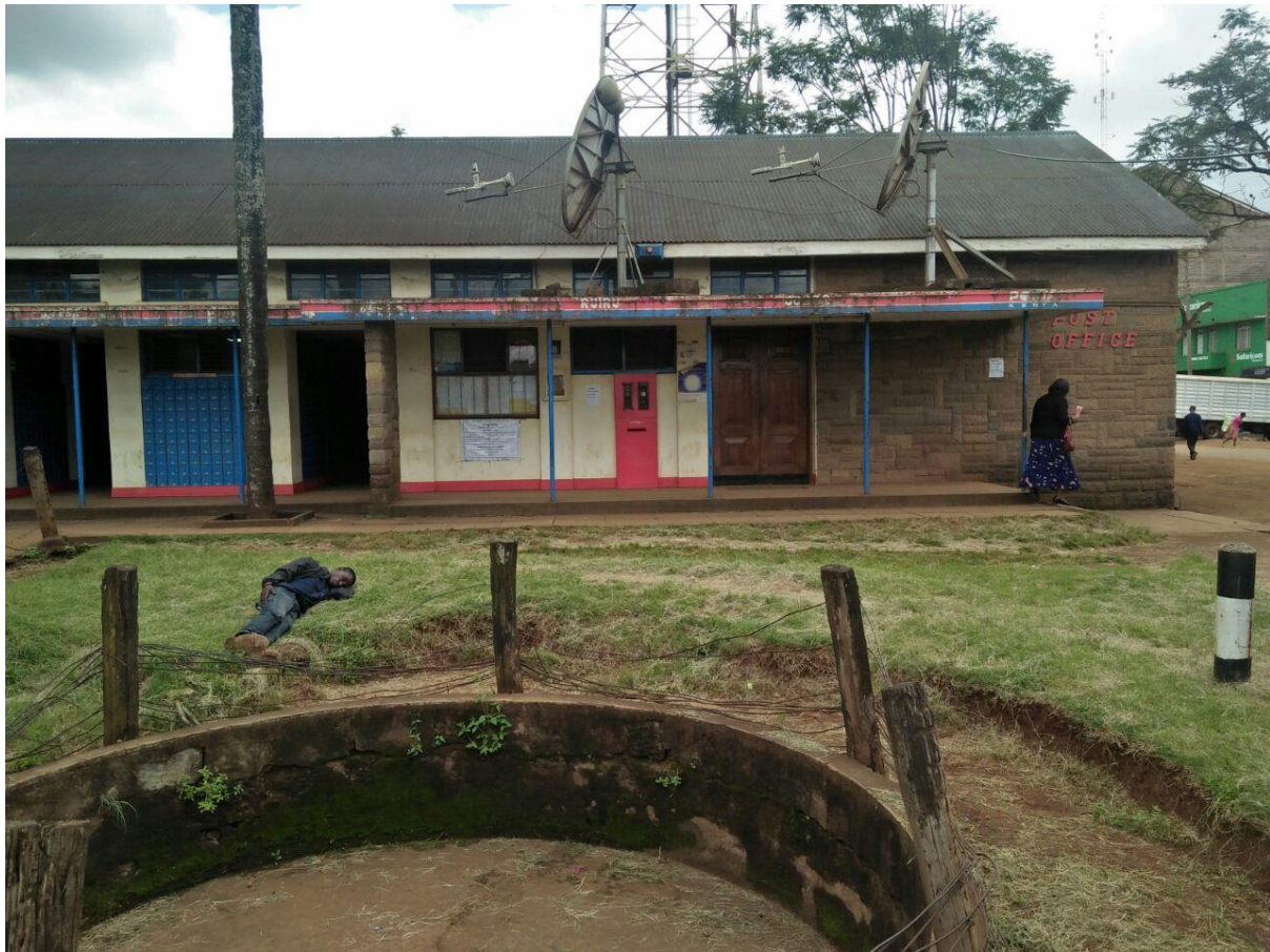
Figure 17: Ruiru Post office located along Biashara Street
