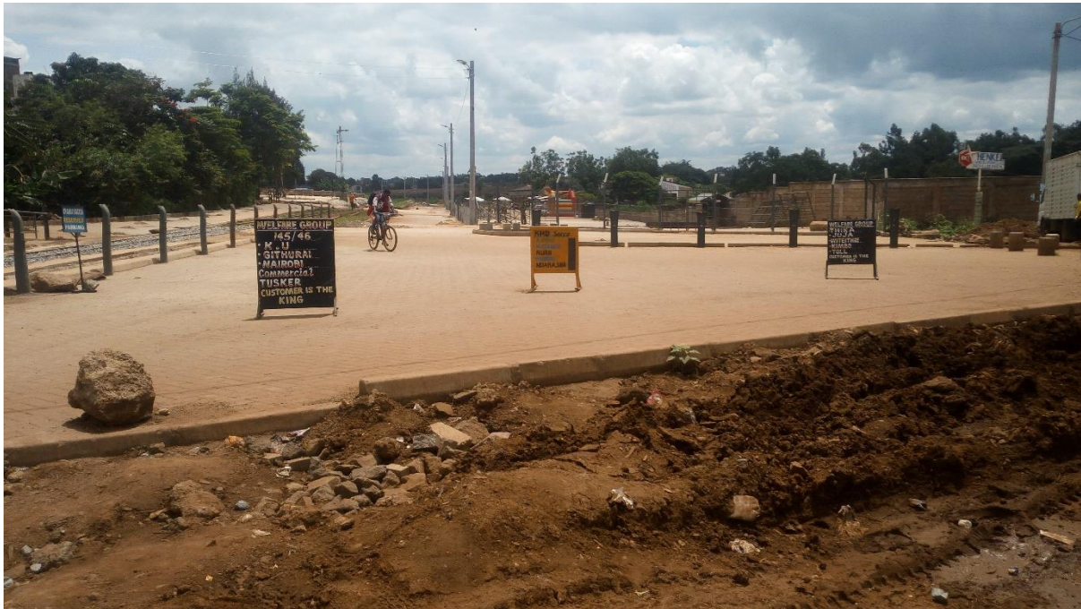
Figure 6: The newly rehabilitated Ruiru Commuter Rail Passenger Terminus
