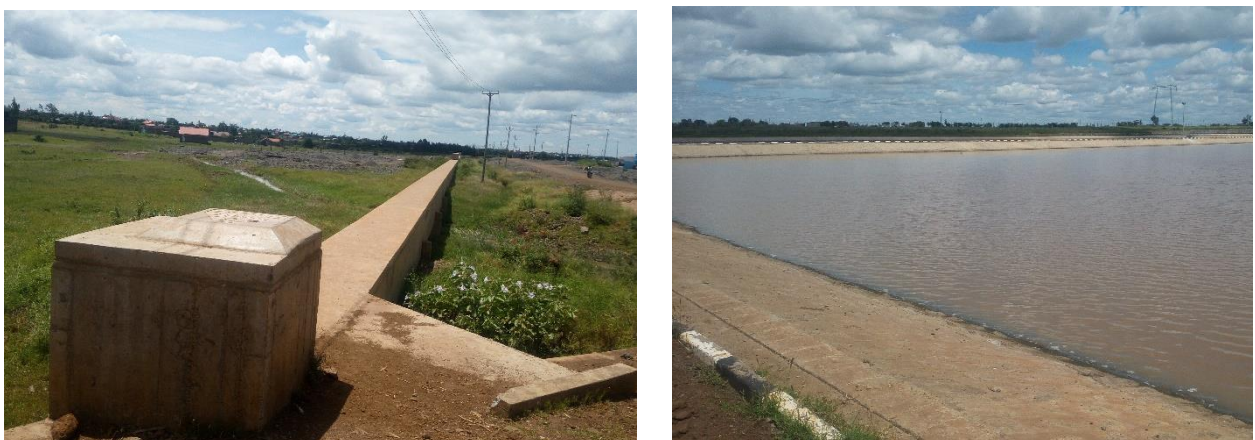
Figure 14: Trunk Sewer to the sewer treatment plant and the waste water treatment plant in Gatong'ora
