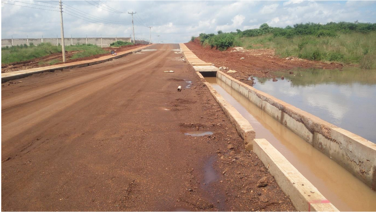
Figure 10: A section of drainage under construction within Tatu City Development
