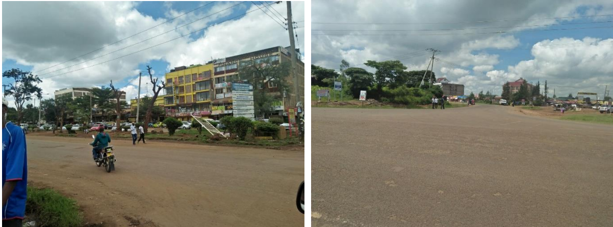
Figure 3: A section of Ruiru-Kamiti Road and the Ruiru-Kamiti Road-Eastern By-pass Junction
