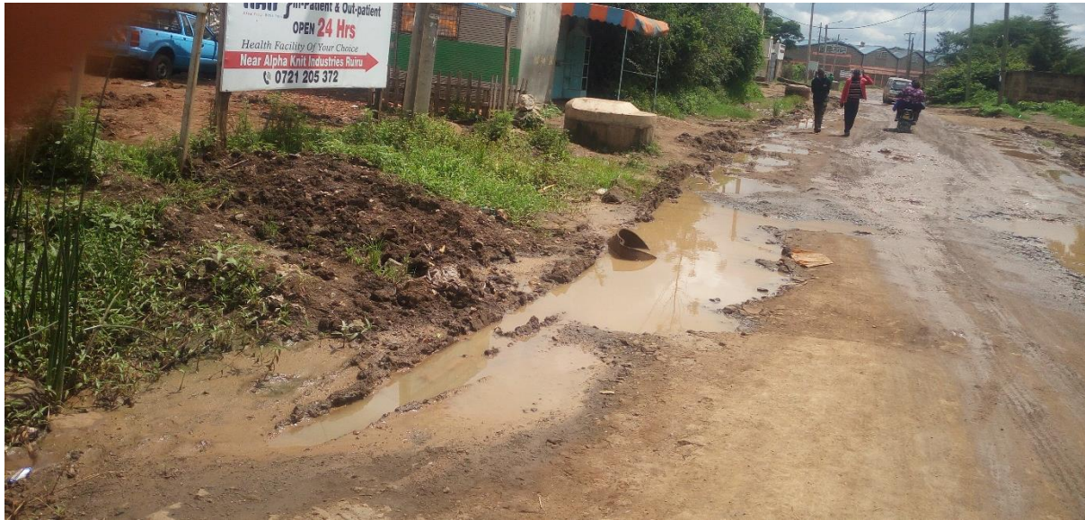
Figure 8: A poorly drained section of a road near Nazareth Hospital
