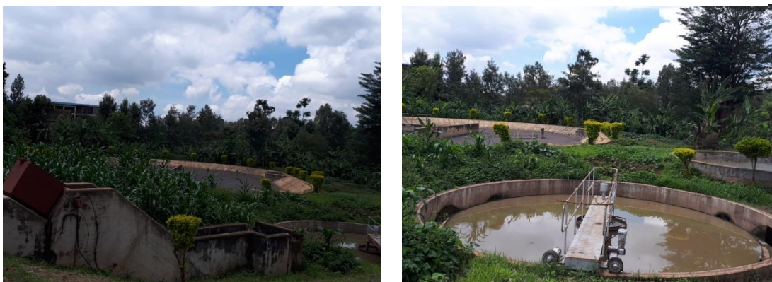
Figure 10: Limuru water and sewerage Project.
