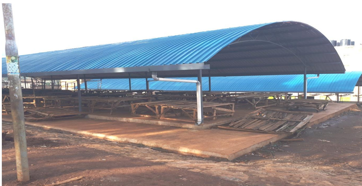
Figure 11: Limuru Market under Construction.
