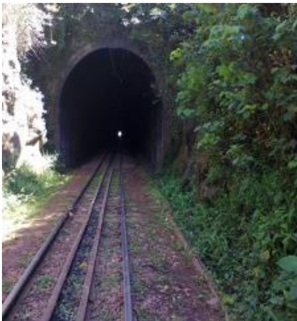
Figure 2: Railway tunnel in Limuru
