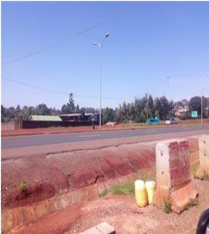
Figure 5: Street lighting along southern bypass Kikuyu
