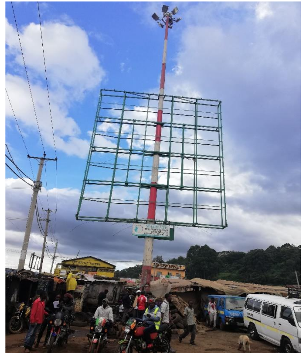
Figure 6: High Mast within Kikuyu Municipality
