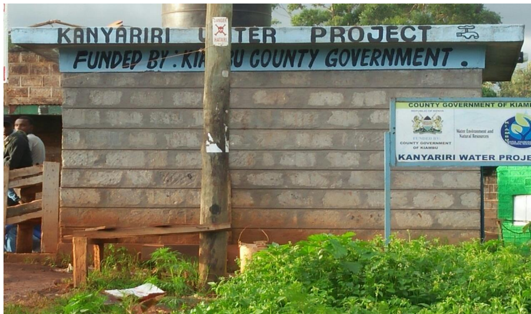
Figure 9: Kanyariri water project funded by the County Government of Kiambu
