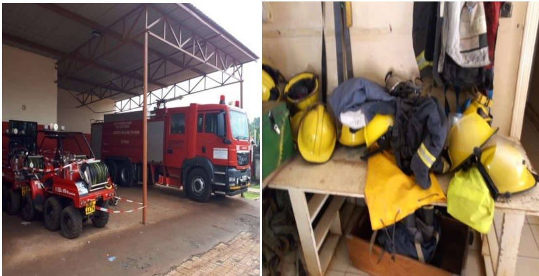
Figure 5: Firefighting Engine and Equipments in Kiambu Fire station.
