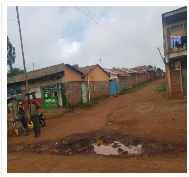
Figure 4 Wega Trading Centre along the Proposed Site
