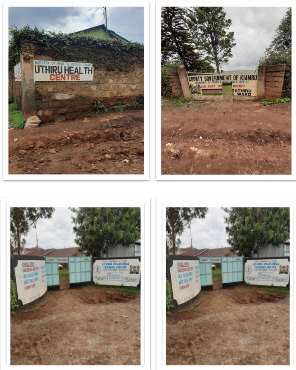
Figure 6 Some of the Basic Infrastructure and Services in the Area
