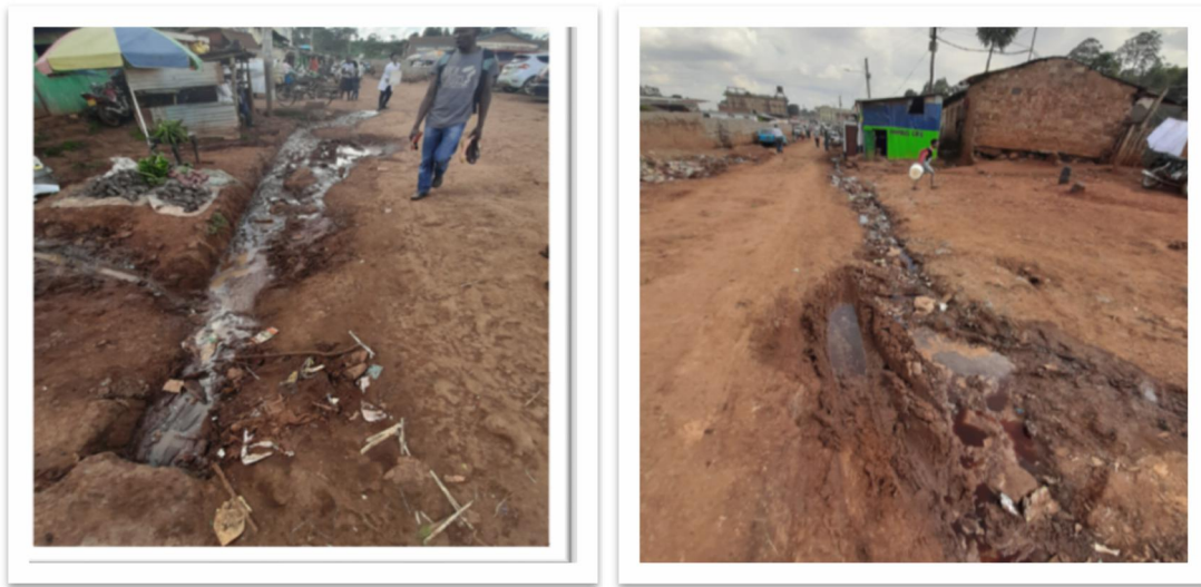
Figure 2 Current Status of the Storm Water Drain in the Project Area
