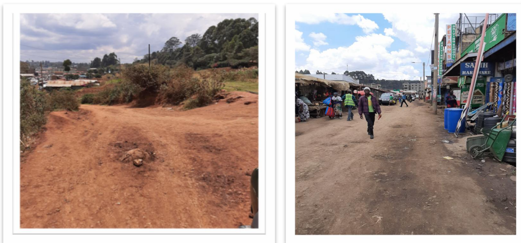
Figure 1 Current Status of the Road in Project Site
