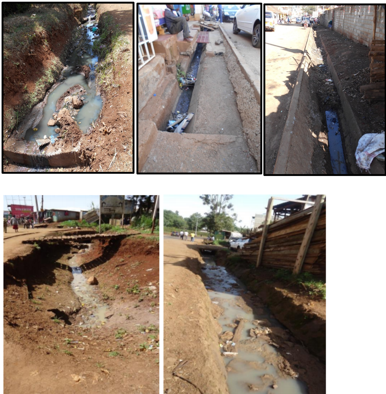
Plate 11: Condition of Storm water drainages
